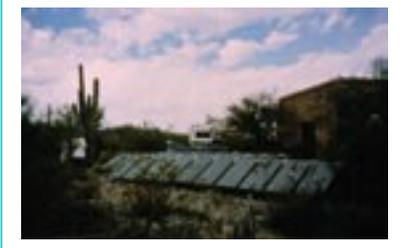
Rural Arizona application of this strategy has been applied to passive water heating (thermosiphon), or for radiant floors. Since hot water rises, and cold water settles, the thermosiphon system has the collector lower than the tank or application. This convective loop runs continuously as the sun shines
