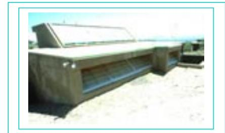
This solar/day lighting element can also include operable windows and glazing to facilitate building natural ventilation exhaust of unwanted interior heat. Now there are four functions for one building element.
