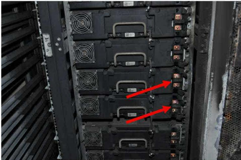
Figure 50 Module power terminals.
