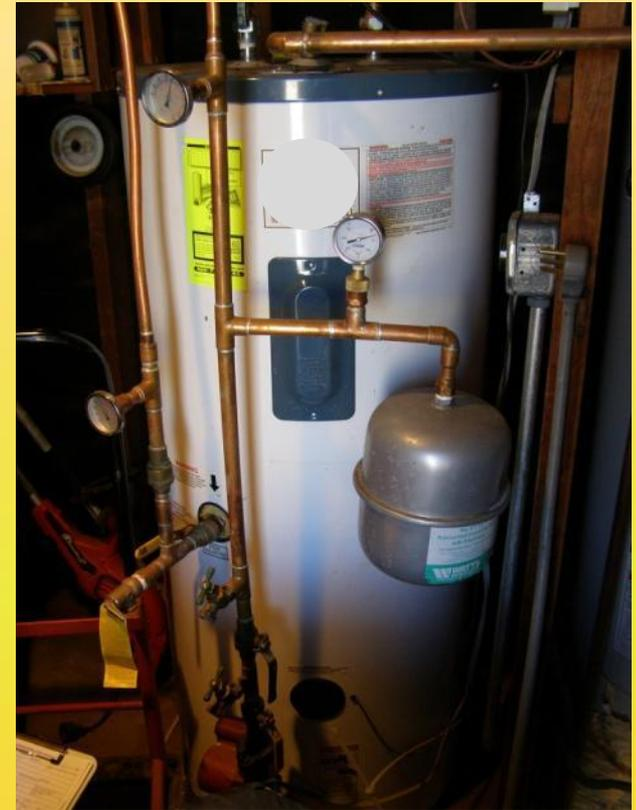
2. Install the EXTROL on the supply side of the boiler, on the suction-side of the heating circulator(s) (see Figure 1).
