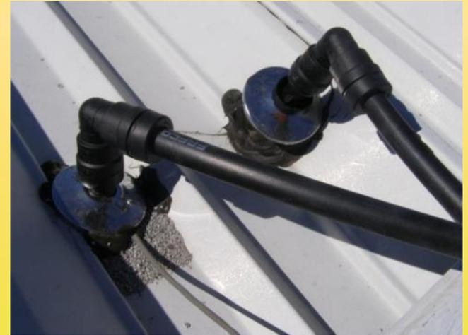
Escutcheons on roof is not an acceptable flashing
