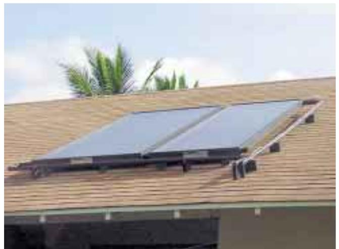
A flat plate solar thermal collector usually consists of copper tubes fitted to a flat absorber plate. The most common configuration is a series of parallel tubes connected at each end by two pipes, the inlet and outlet manifolds. The flat plate assembly is contained within an insulated box, and covered with low-iron, tempered glass. (See the diagram on page 45.)
