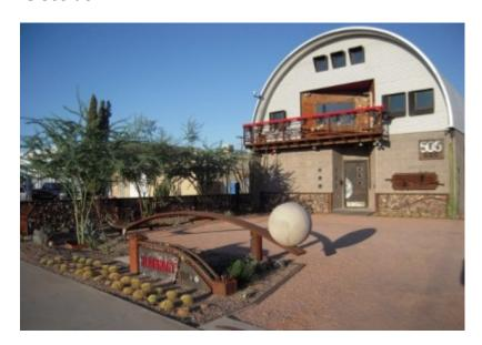
Completed in 2008, the studio is constructed from glass and steel, and a vast amount of additional material in this project are used or recycled. The Studio is 3,700+ sf with 28 foot ceilings. Beautiful natural light pours through the 7 skylights and north windows.
