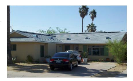
This House was built in 1961 — the era of cheap energy, and the insulation and mechanical system equipment reflected it. There was no wall insulation, just masonry block and single pane windows and HVAC equipment with a SEER rating of about 8 located on the roof, with the leaky duct work running through the hot attic. This is the typical situation found in the existing inventory of homes in the valley. An attic fire provided the opportunity for a complete remodel.
