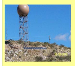
Argent used excavators and jack-hammers to dig fourteen, 4 foot deep core footings along 100 feet of hillside to secure the photovoltaic panel mounting structure. Incredibly, the construction was completed in 14 days and the solar power system is now in operation.
